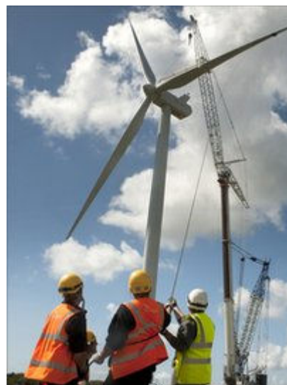
The last of the six replacement turbines are now in place
